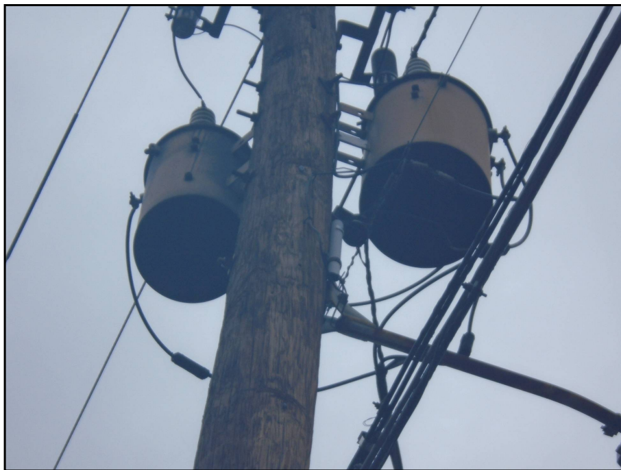
24 : View of a typical pole-mounted electrical transformer
